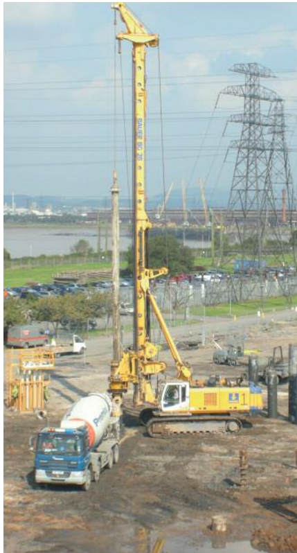
Pile installation with one of the BG28 drilling rigs
